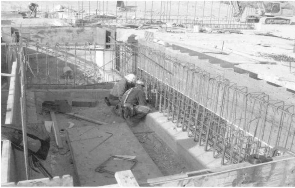
*Don Ponciano (left) & Josh Triner (right) tie in rebar on an exterior wall ...creating a "cage" of reinforcement for the concrete wall.*
